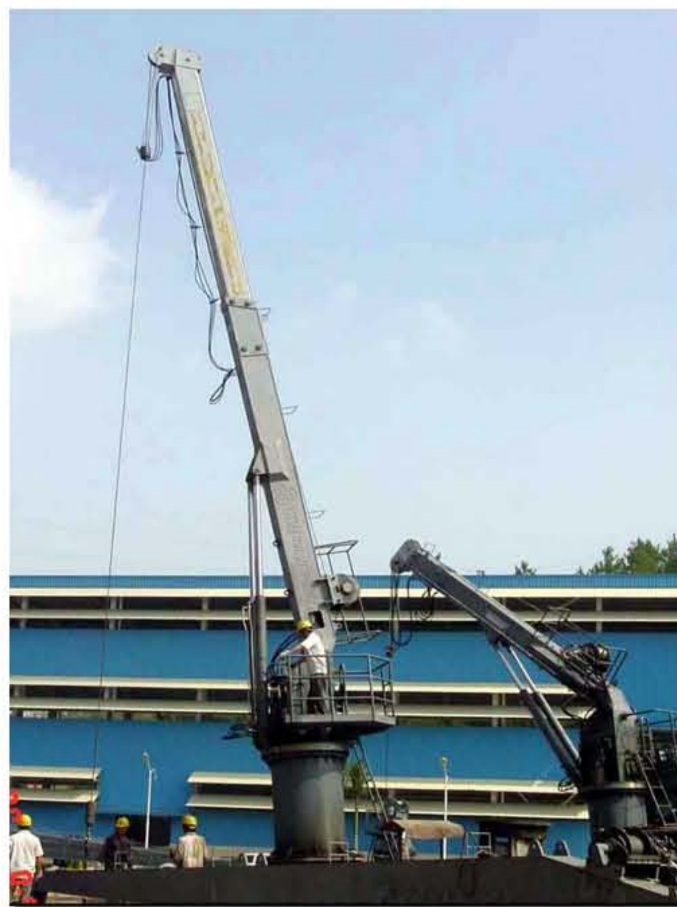
SCM Crane Testing
